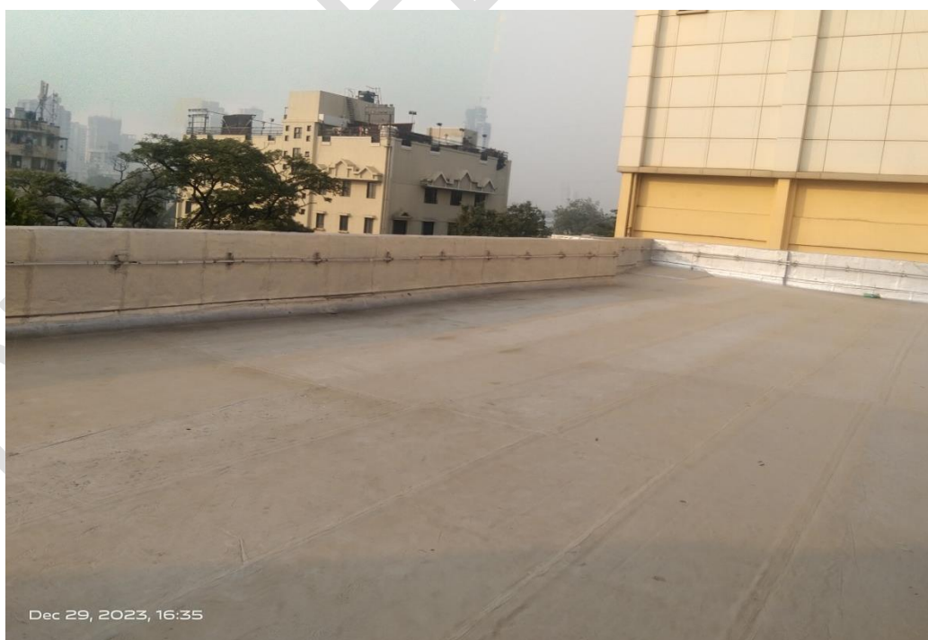
Plate 8: Recently fabricated rooftop that reflects the harsh sun rays
